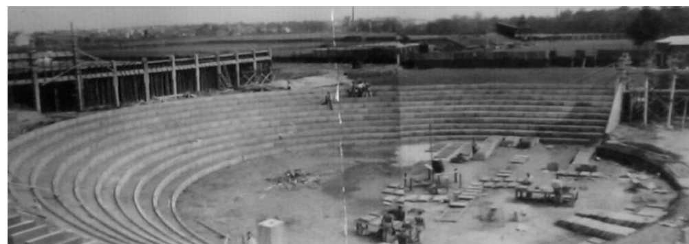
Photo B: Construction of the amphitheatre during the 1930s (object 1)
